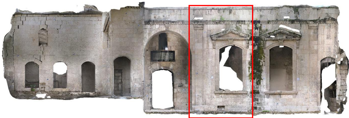
Figure 116: Stone-by-stone surveying (Total Station)
